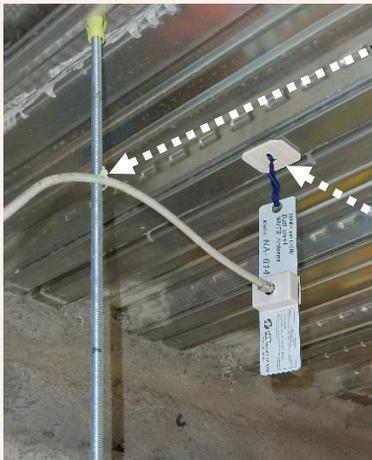
Tie the coax cable to the hanging bolt with using cable tie.
